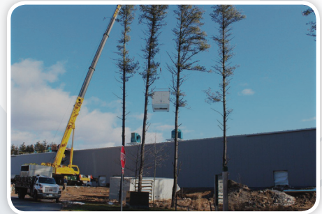
A 275 ton crane lifts one of the massive rooftop HVAC units into place at 20 Tech Trail.
